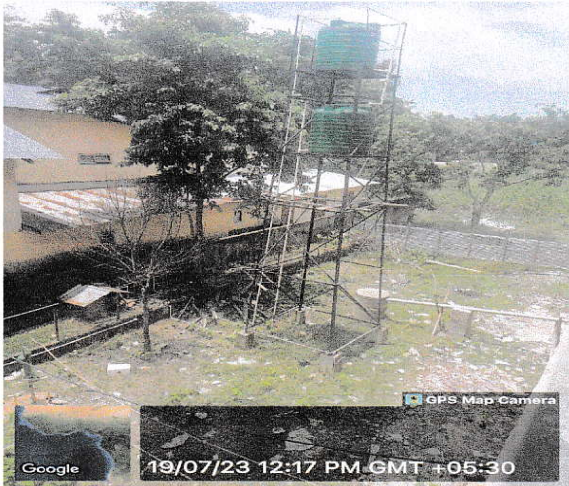
Over Head Water Tank
